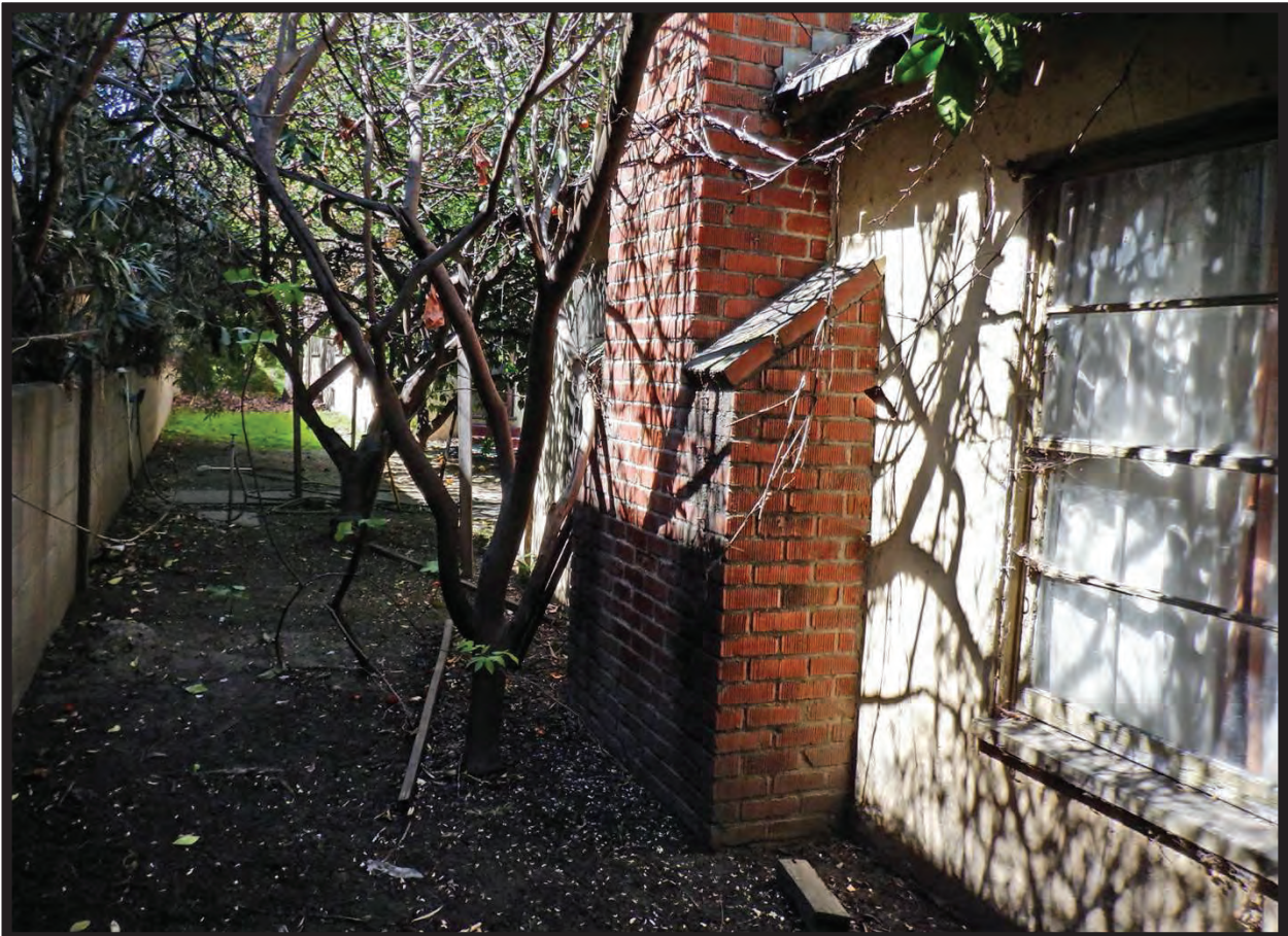
South Elevation of 1944 Residence at 1022 La Cadena Avenue, Arcadia, CA (WNW)
