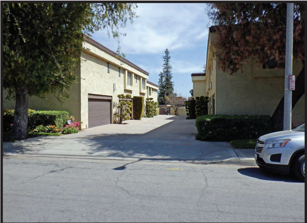
Residences at 1102 La Cadena Avenue, Arcadia, CA (MFR, 1974; E)
