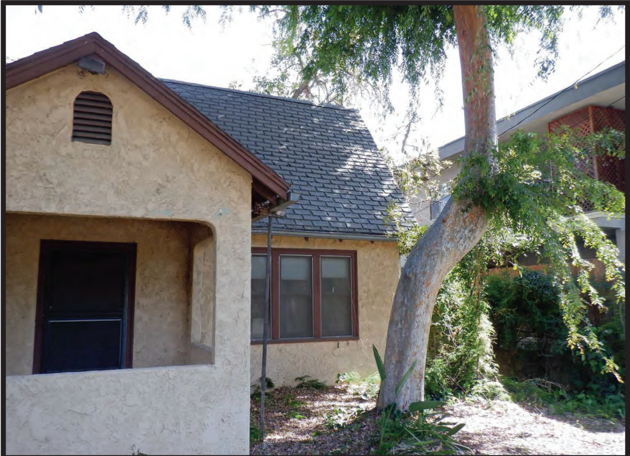
West Elevation of Residence at 1022 La Cadena Avenue, Arcadia, CA (ESE)
