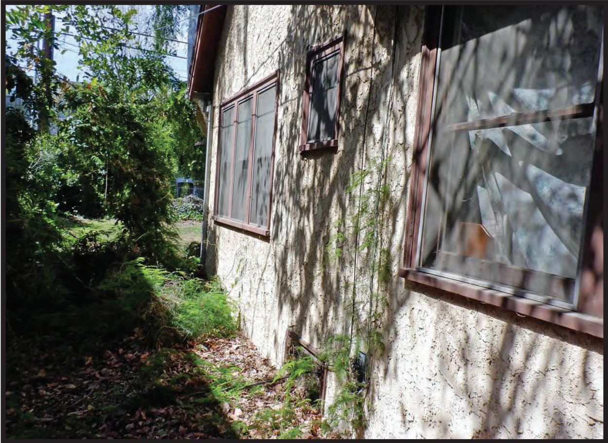
South Elevation of Residence at 1022 La Cadena Avenue, Arcadia, CA (WNW)
