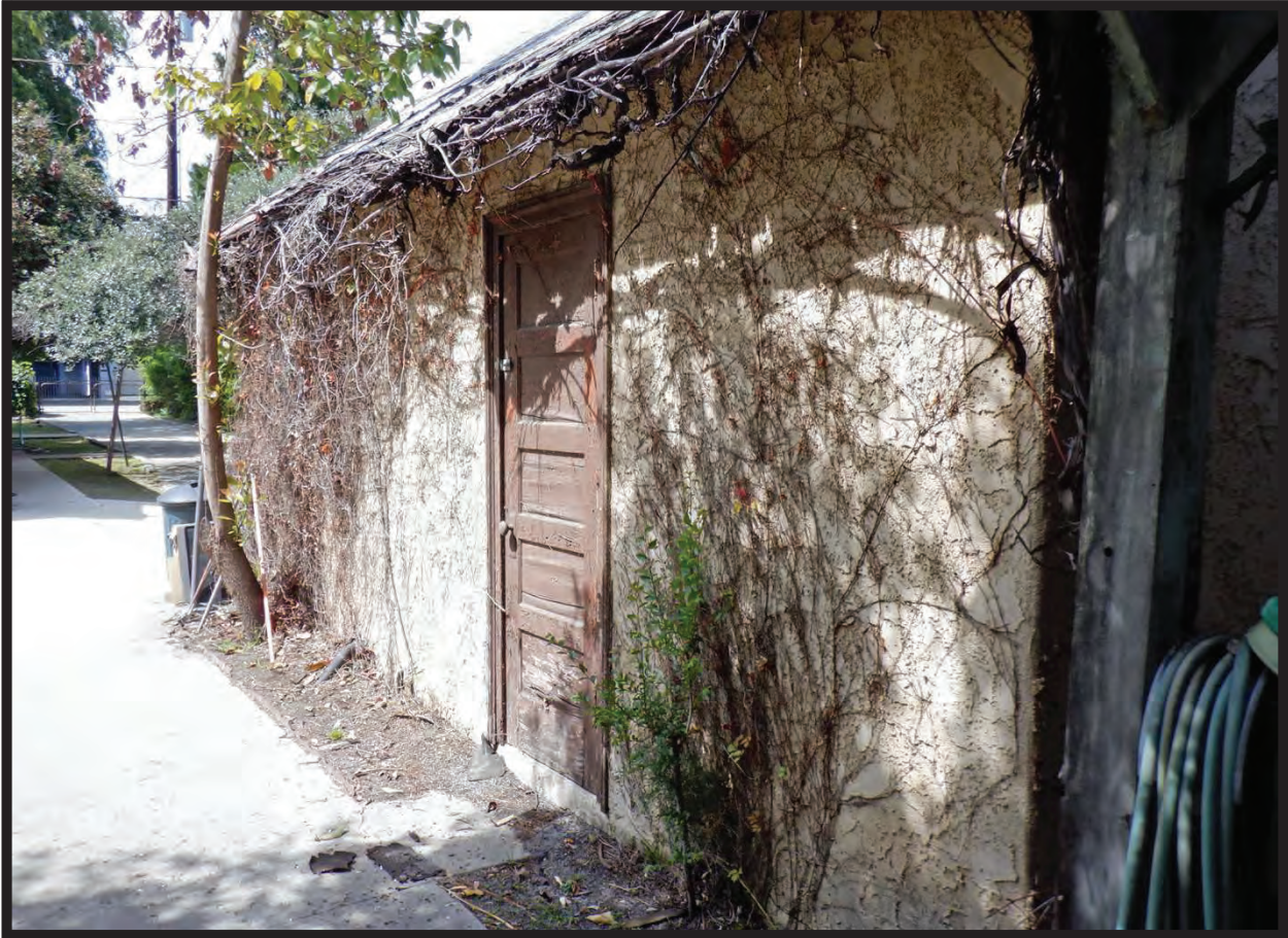
South Elevation of 1926-1927 Garage, 1022 La Cadena Avenue, Arcadia, CA (WNW)
