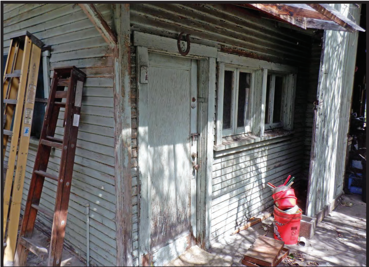
Western End of Large Barn/Workshop, 1022 La Cadena Avenue, Arcadia, CA (NE)
