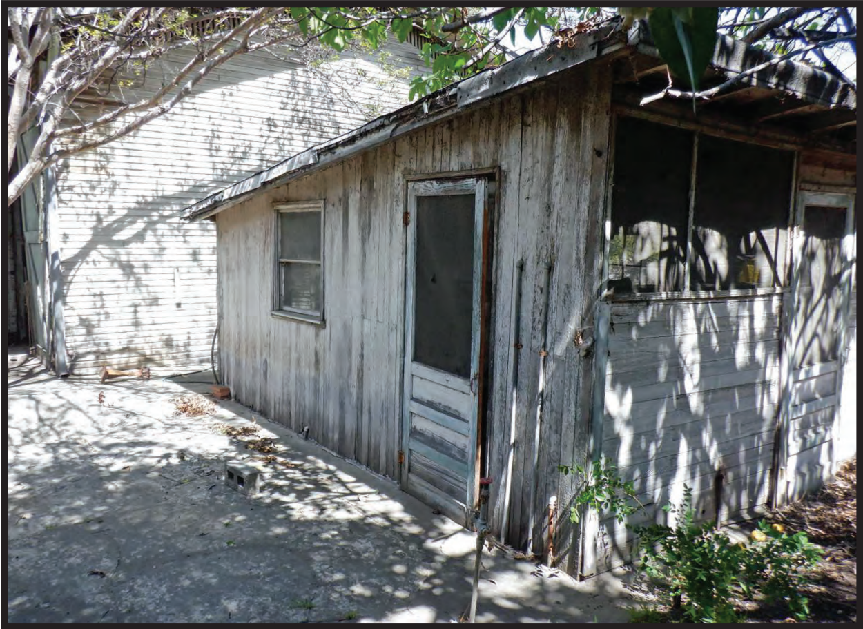
Shed East of 1944 Residence at 1022 La Cadena Avenue, Arcadia, CA (NE)
