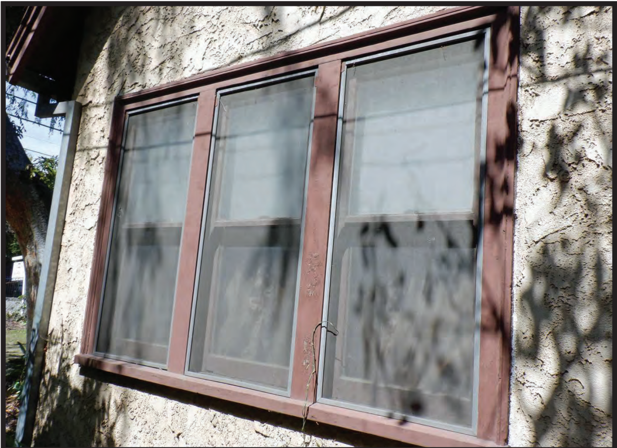
Window Detail, South Elevation of Residence at 1022 La Cadena Avenue, Arcadia, CA (NW)
