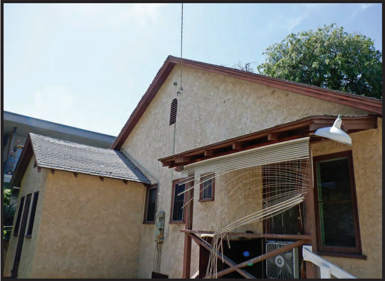
East Elevation of Residence at 1022 La Cadena Avenue, Arcadia, CA (SW)
