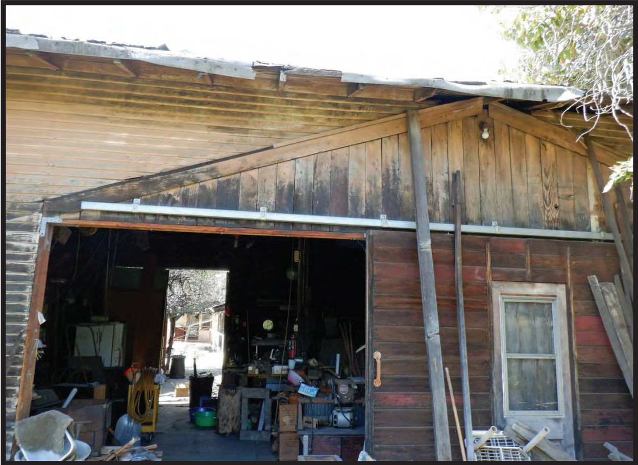
East Elevation of Large Barn/Workshop, 1022 La Cadena Avenue, Arcadia, CA (W)
