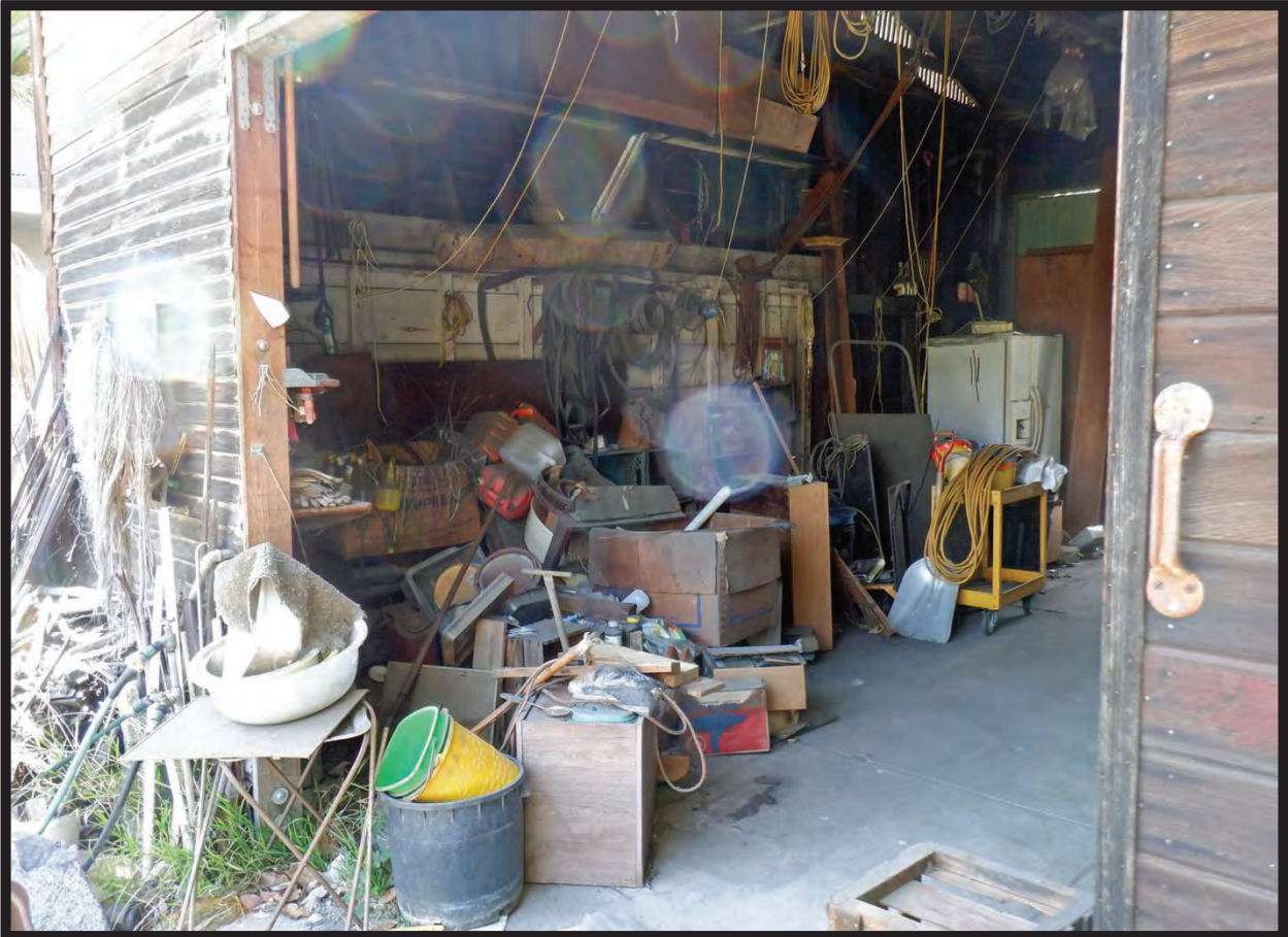
Detail, East Elevation of Large Barn/Workshop with Bay Door, 1022 La Cadena Avenue, Arcadia, CA (WSW)
