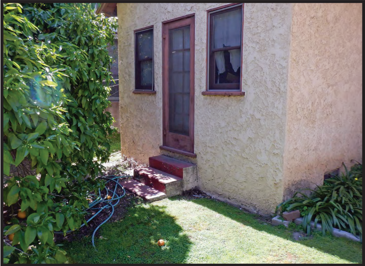
Entrance on Addition, East Elevation of Residence at 1022 La Cadena Avenue, Arcadia, CA (SW)
