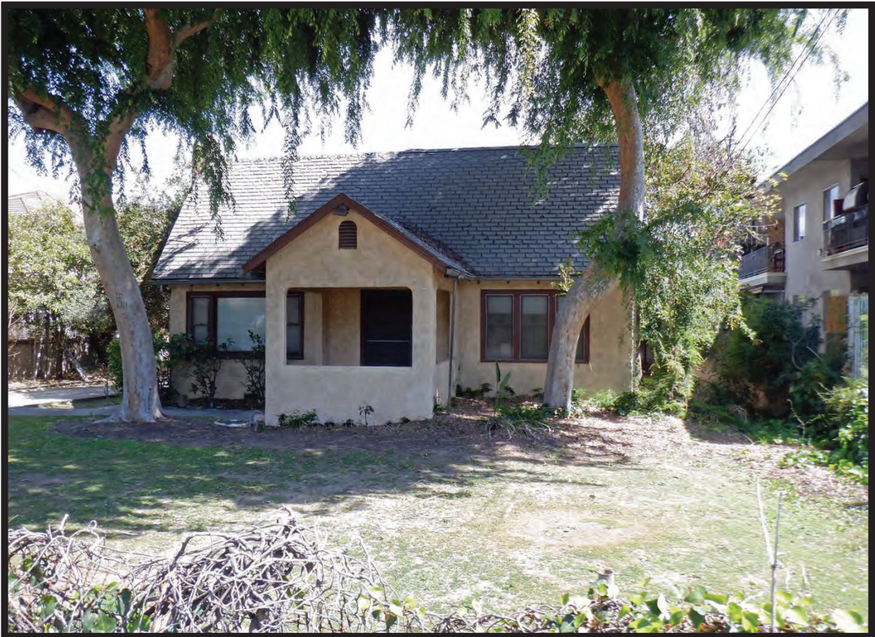
West Elevation of Main Residence at 1022 La Cadena Avenue, Arcadia, CA (MFR, 1926-1927; E)
