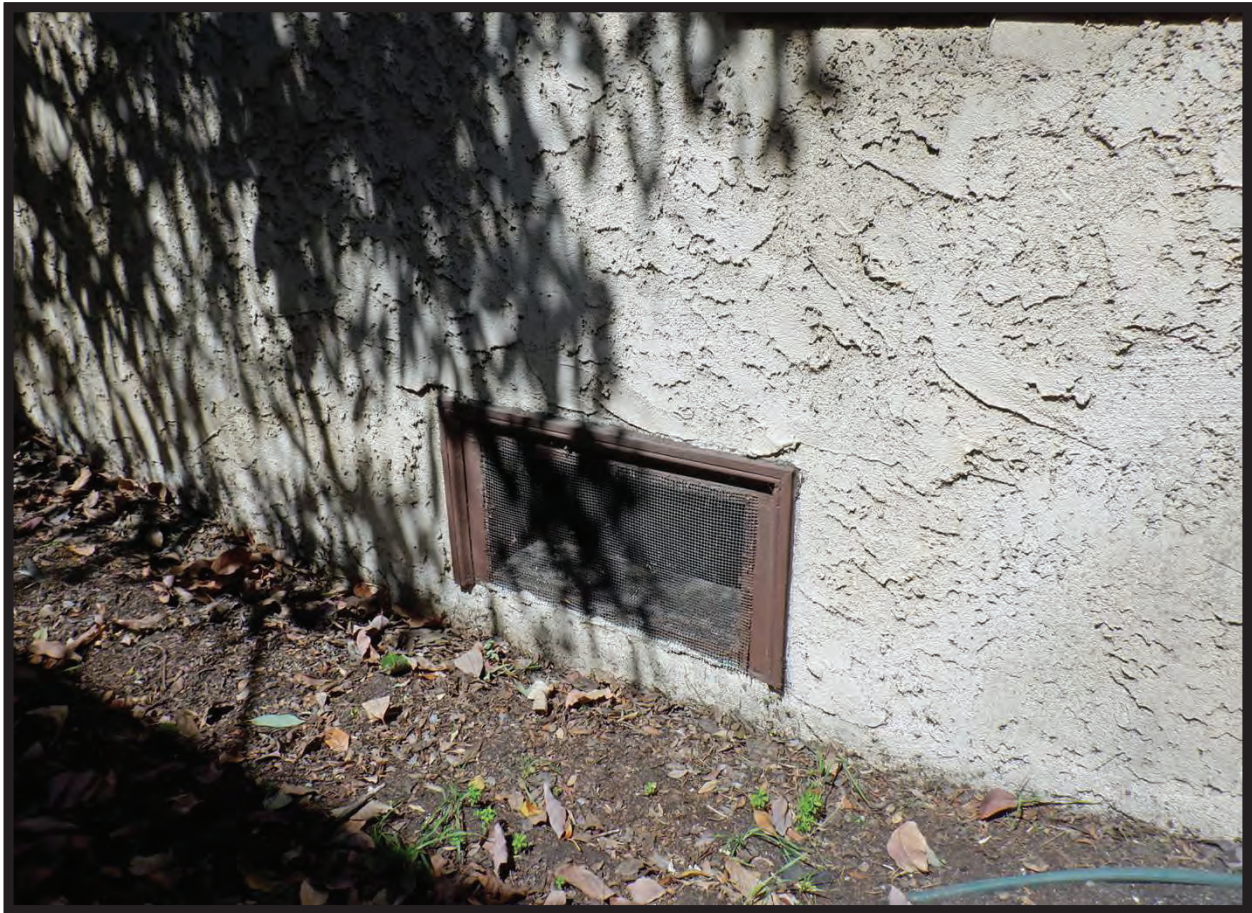
Crawl Space Entry, South Elevation of Residence at 1022 La Cadena Avenue, Arcadia, CA (NW)
