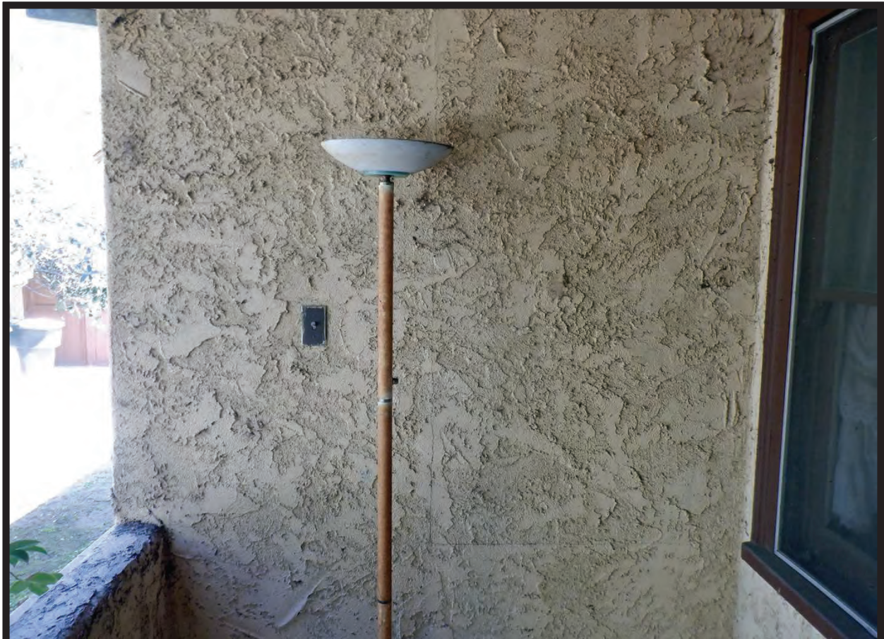
Wall Detail, Side Porch, North Elevation of Residence at 1022 La Cadena Avenue, Arcadia, CA (E)
