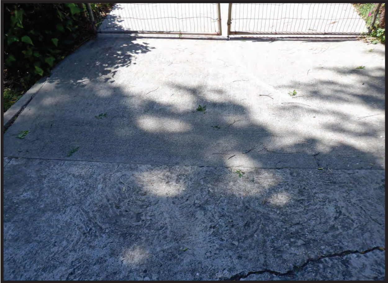
Detail of Driveway Pavements, 1022 La Cadena Avenue, Arcadia, CA (W)
