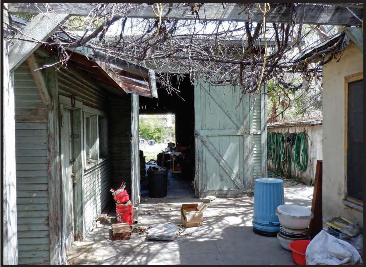
Office and West Elevation of Barn/Workshop, 1022 La Cadena Avenue, Arcadia, CA (E)
