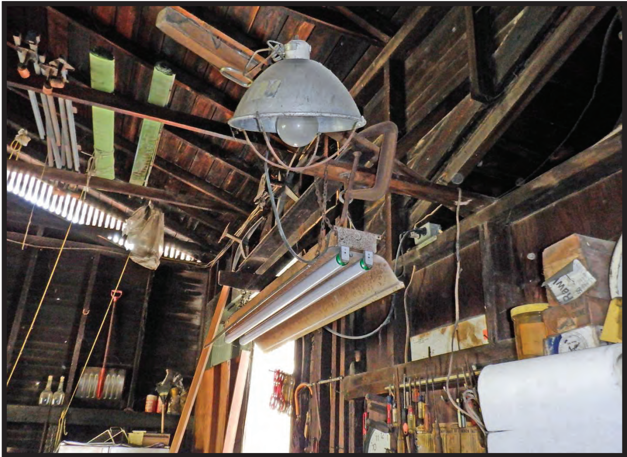
Interior Detail, Large Barn/Workshop with Bay Door, 1022 La Cadena Avenue, Arcadia, CA (SSW)
