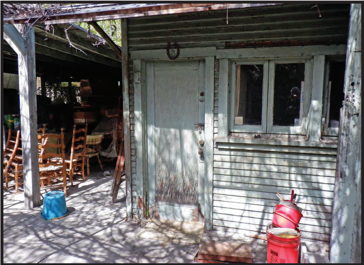
South Elevation of Western End of Large Barn/Workshop, 1022 La Cadena Avenue, Arcadia, CA (NNW)
