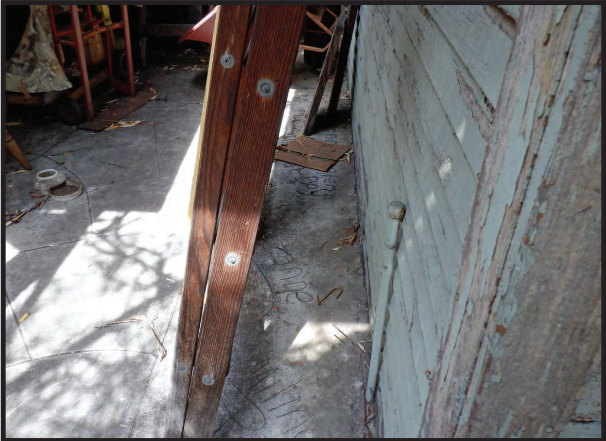
Markings in Concrete to West of Office, 1022 La Cadena Avenue, Arcadia, CA (Detail)
