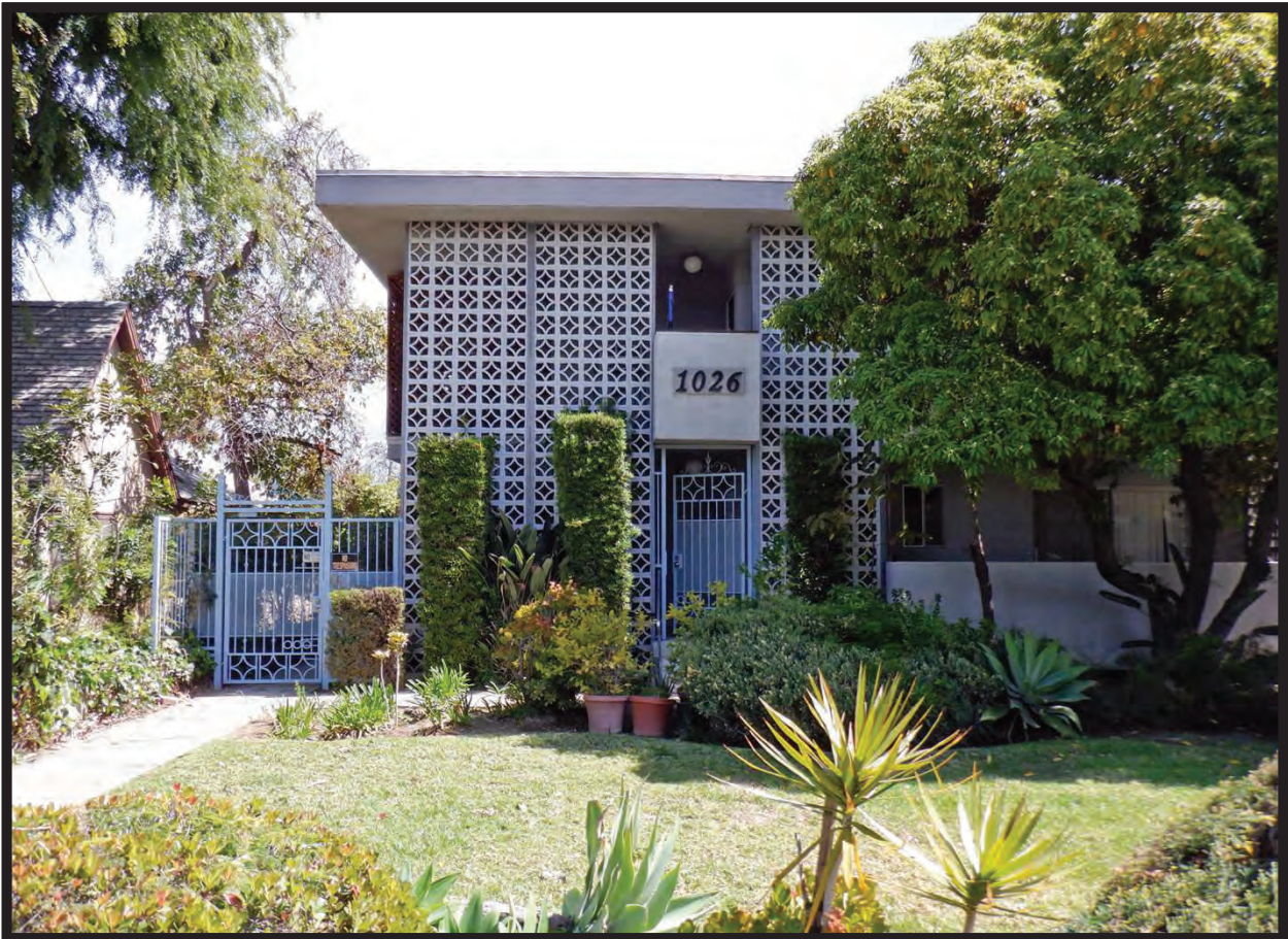
Residences at 1026 La Cadena Avenue, Arcadia, CA (MFR, 1964; E)
