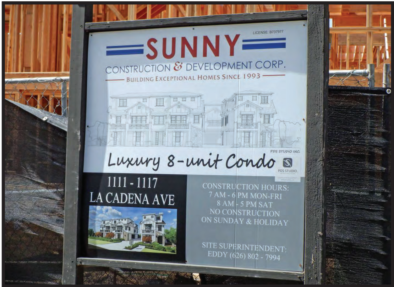
Signage at Construction Site, Arcadia, CA.
