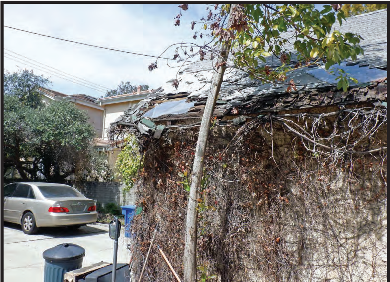
South Elevation of 1926-1927 Garage, 1022 La Cadena Avenue, Arcadia, CA (NW)
