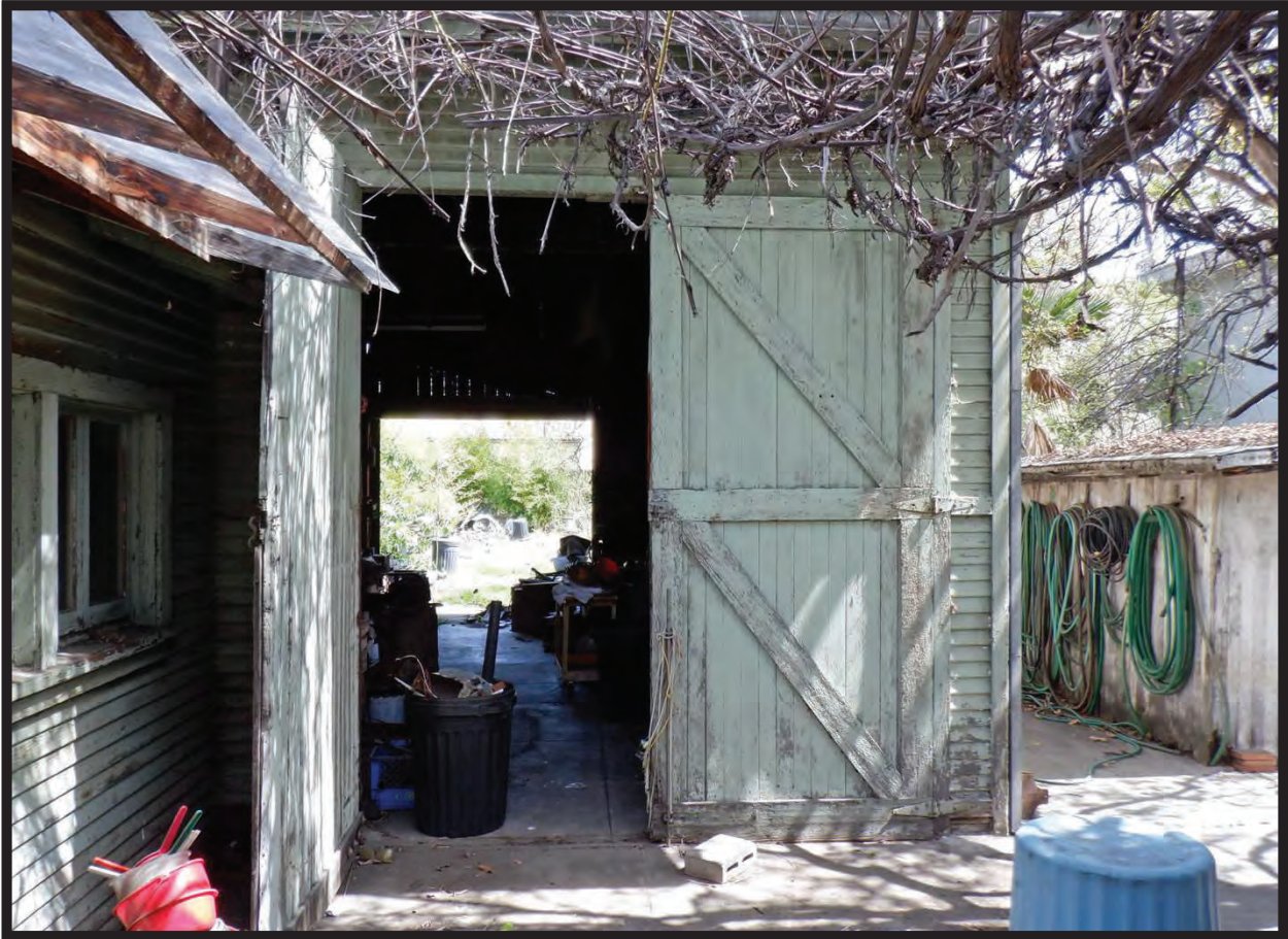
West Elevation of Large Barn/Workshop, 1022 La Cadena Avenue, Arcadia, CA (E)
