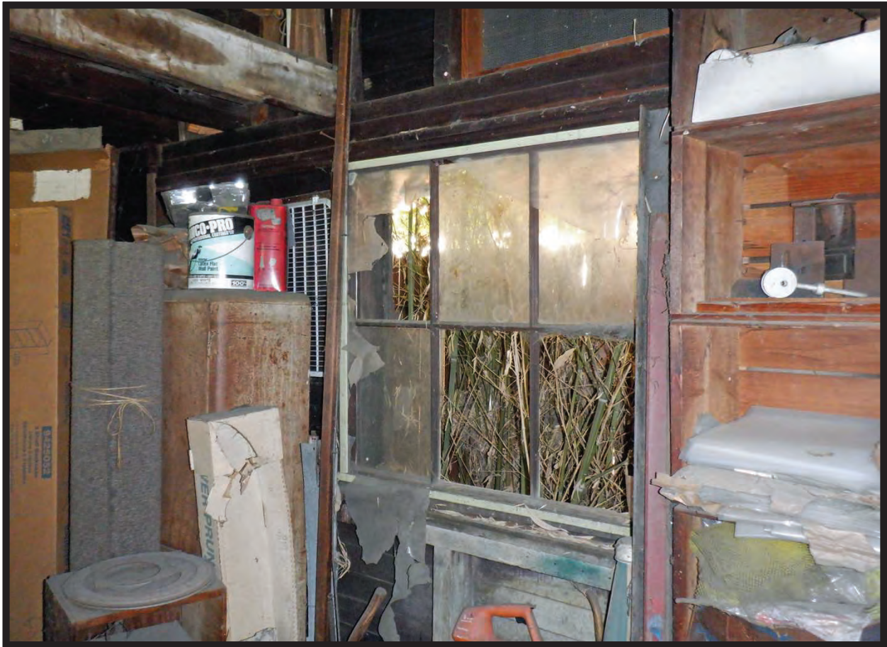
Interior Detail, Large Barn/Workshop with Bay Door, 1022 La Cadena Avenue, Arcadia, CA (NNW)
