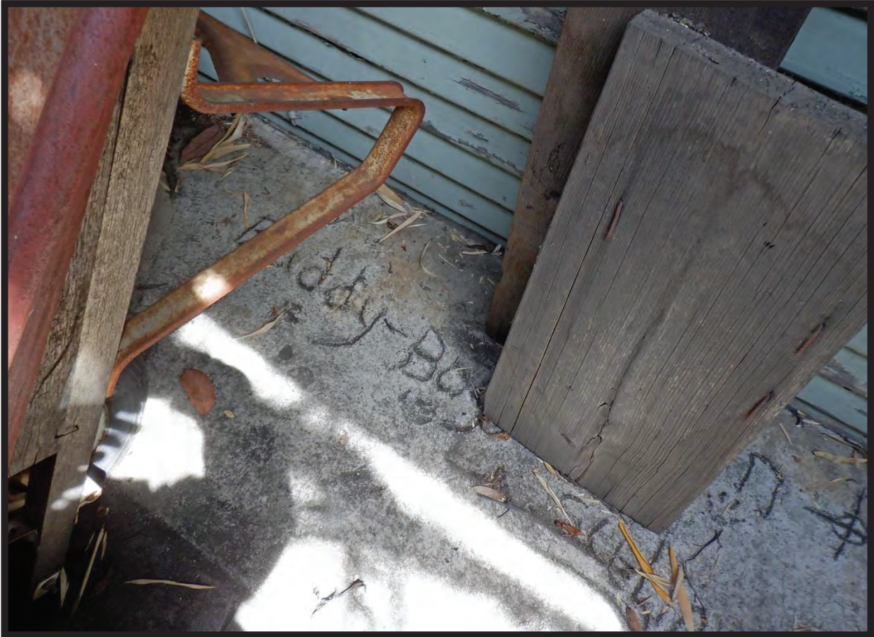
Markings in Concrete to West of Office, 1022 La Cadena Avenue, Arcadia, CA (Detail)
