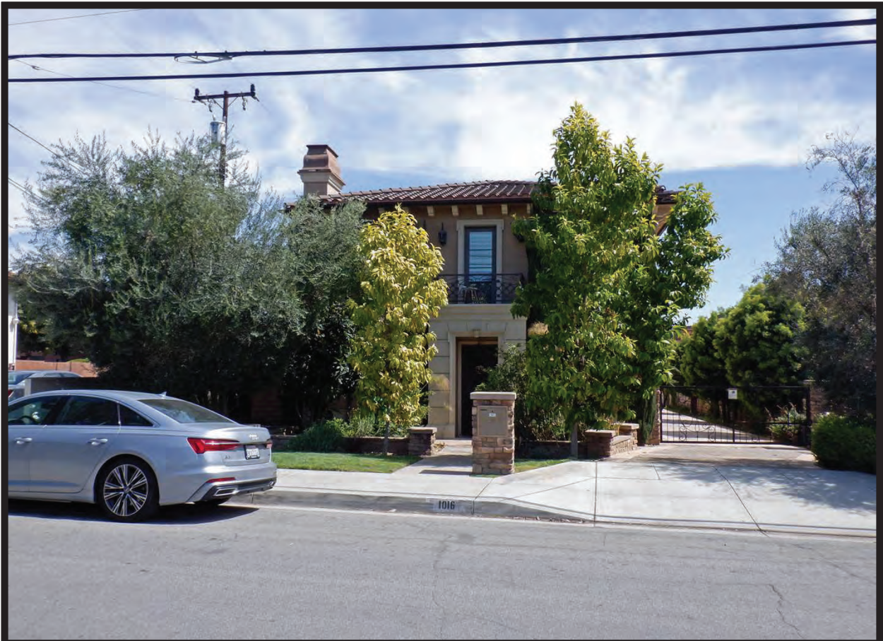
Residences at 1016 La Cadena Avenue, Arcadia, CA (MFR, 20011-2012; E)
