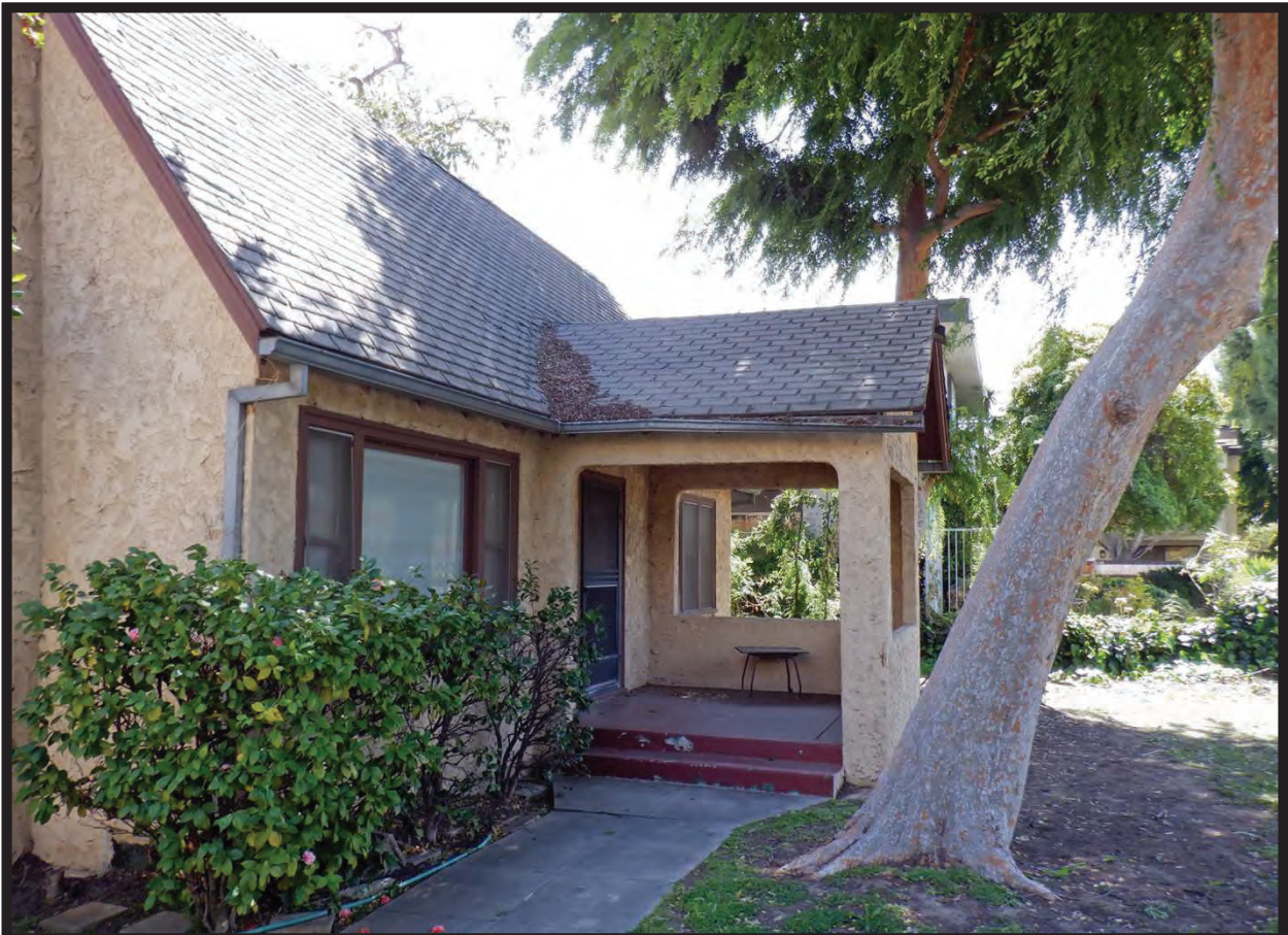
West Elevation of Residence at 1022 La Cadena Avenue, Arcadia, CA (SSE)
