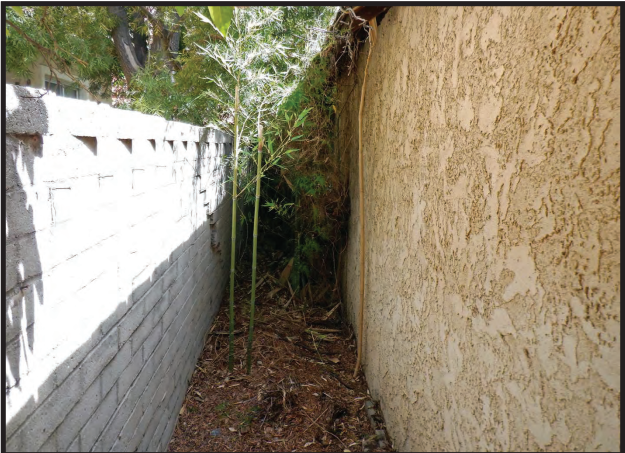
Northern Property Boundary along 1926-1927 Garage, 1022 La Cadena Avenue, Arcadia, CA (E)
