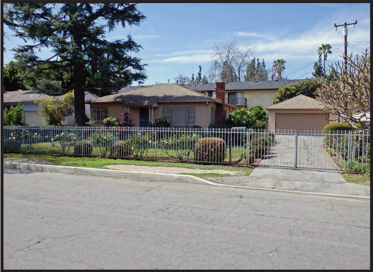
Residence at 1011 La Cadena Avenue, Arcadia, CA (SFR, 1951; WSW)
