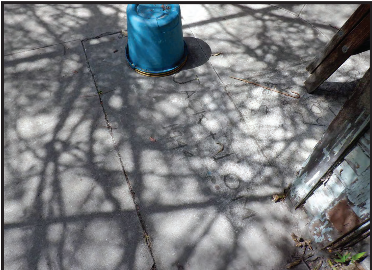
Markings in Concrete to West of Office, 1022 La Cadena Avenue, Arcadia, CA (Detail)
