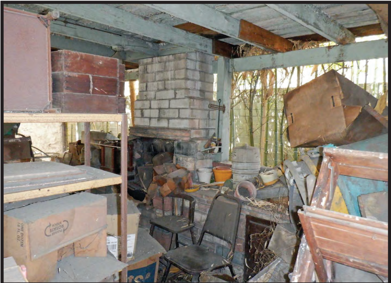
Covered Patio between Office and Garage, 1022 La Cadena Avenue, Arcadia, CA (NW)
